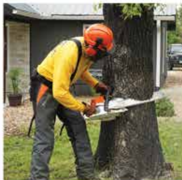
Cut and remove fallen trees and limbs on homes after tornadoes.
